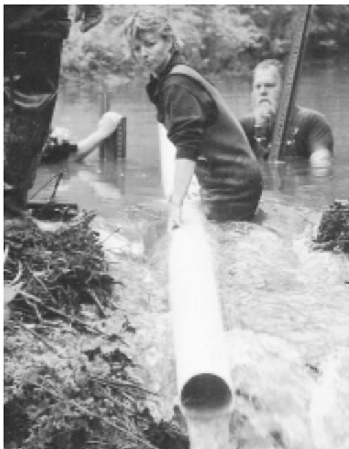
PVC pipes can be run through beaver dams to control flooding problems and to deceive beavers who don't realize that their dam has been breached. Above, Deb Gode installing pipes with the Army Corps of Engineers in Tennessee.
